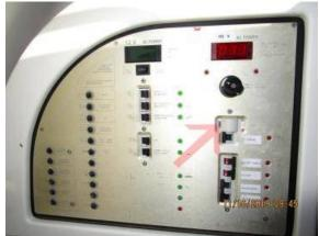
**A.C. power selector switch:** AC/Generator manual break/make lever switch located in main AC panel.
